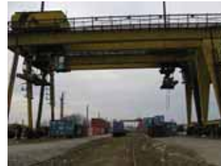
Container terminal for use by railroad, in Bucharest
