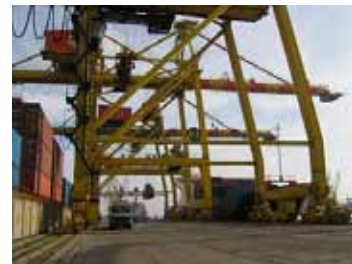
At the existing container terminal in the North Port
