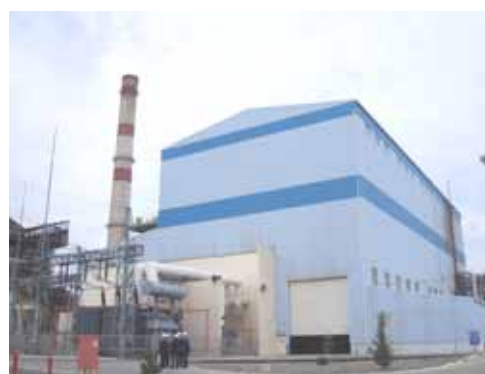
Severnaya Gas Combined Cycle Power Plant
