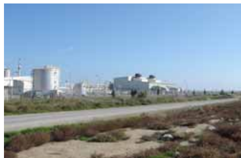
Karadakh Gas Compressor Station
