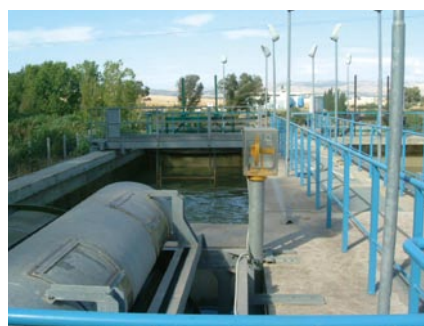
Water supply facility
