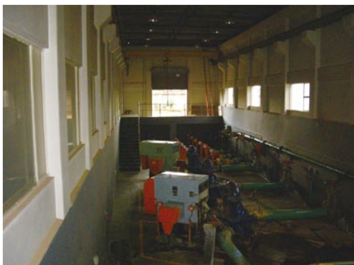
Inside a water purification facility
