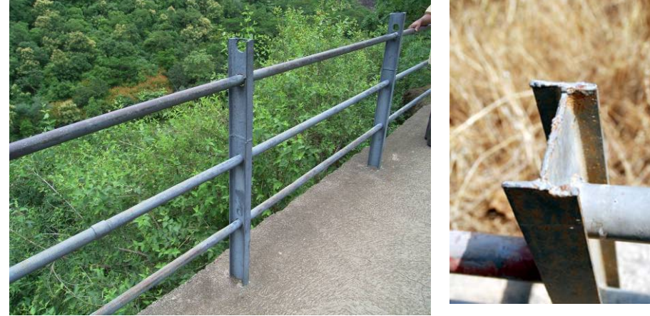
(Figure 14) Guardrail built with H-shaped steel rods
