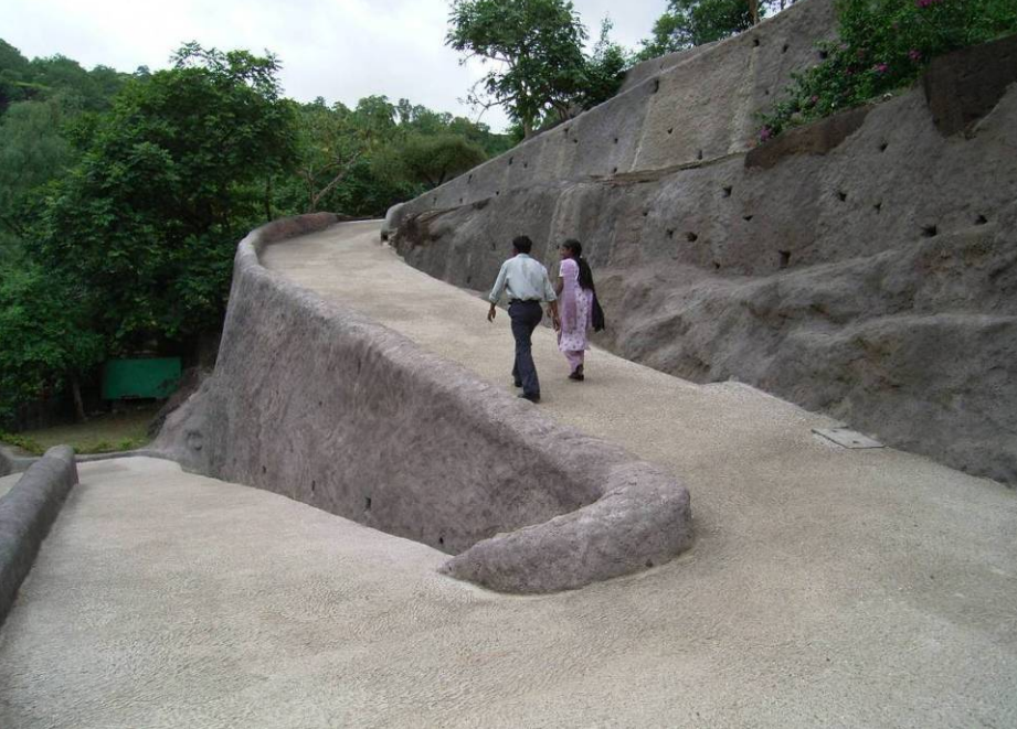
(Figure 13) Newly constructed slopes and slope surface which has been sprayed with cement to artificially create an appearance of rock surface
