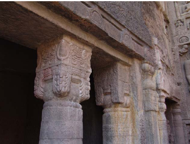
(Figure 27) Reconstructed column capitals (left) and original column capitals (right) in the right shrine at cave 19
