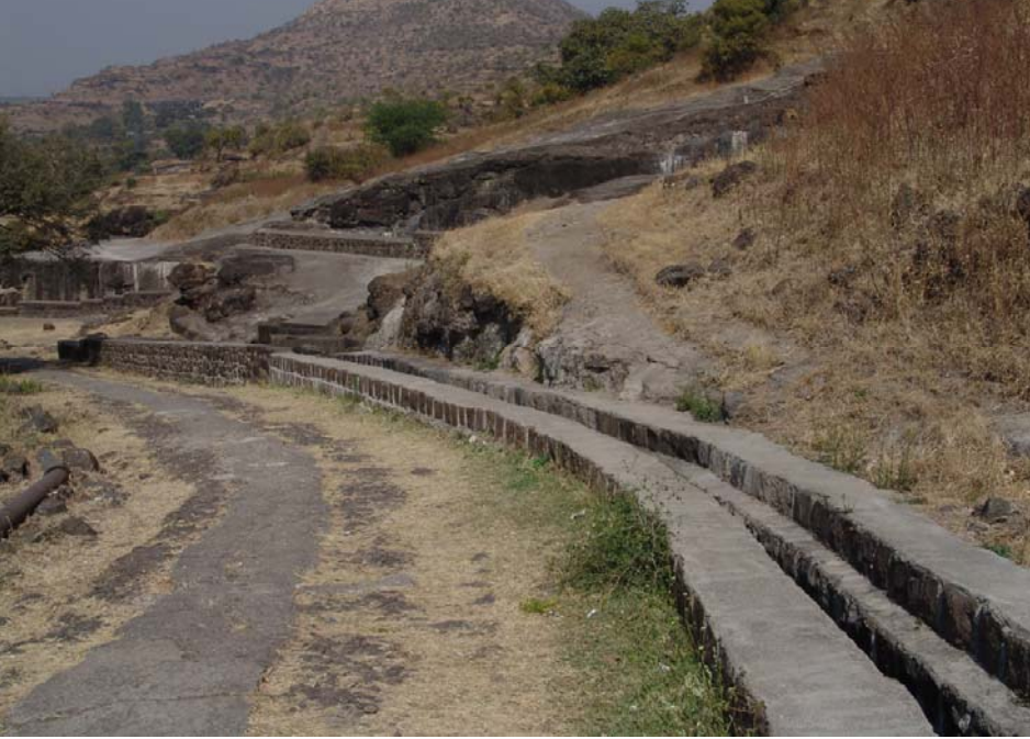
(Figure 49) Drainage maintenance work Above cave 16(left), drainage system carrying water from above cave 1 to side of cave 16
