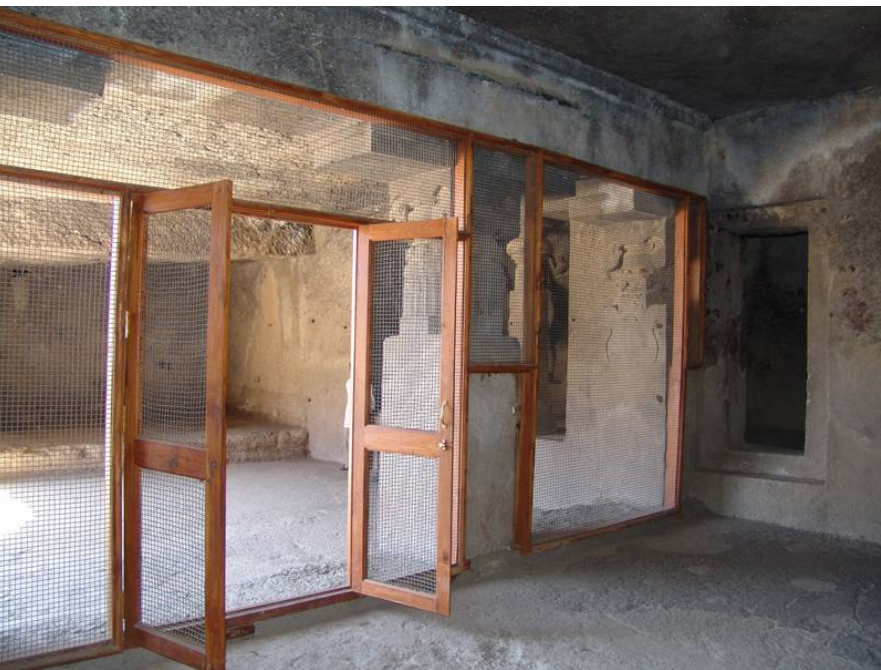
(Figure 51) Installation of bat proof mesh Cave 5 (above and below)
