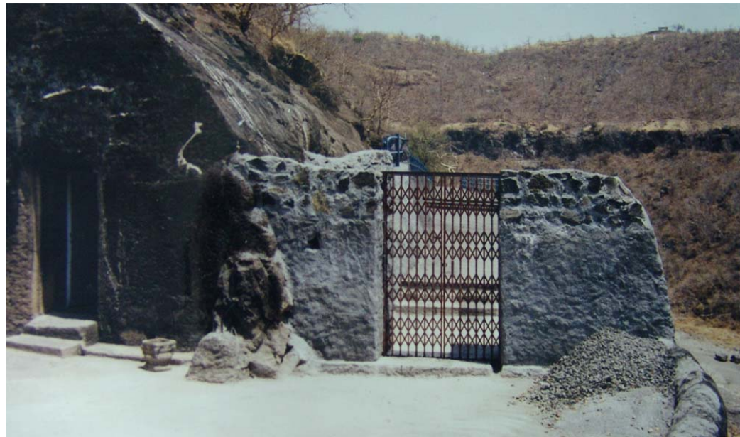
(Figure 59) Gate at Ajanta historic site with surface artificially made to appear like natural rock
