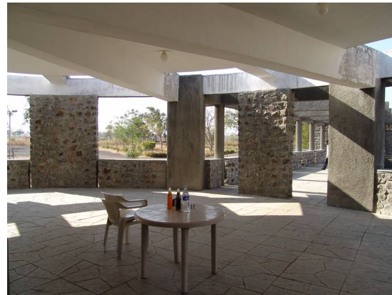
(Figure 71) Restaurant built at Viewpoint
