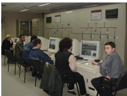
Control room at a thermal power plant (Azerbaijan)
