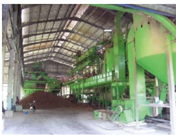
Palm oil plant supported by a sector loan (Thailand)
