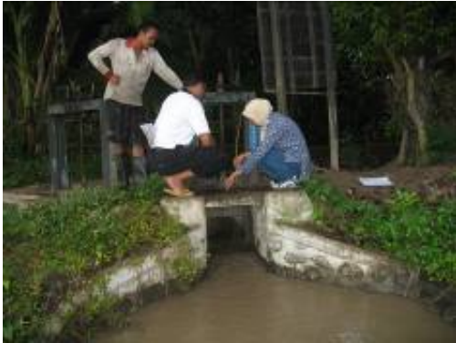
Gate control works by P3A (Water Users Association) staff at a tertiary canal
