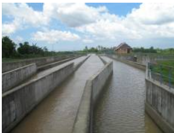
Completed Primary Irrigation Canal of Bissua Irrigation Scheme
