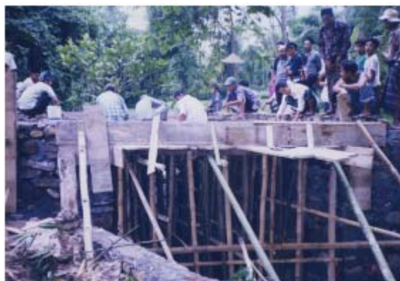
Tertiary irrigation canal (South Sulawesi) & bridge (West Nusa Tenggara) under construction by local communities
