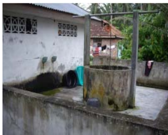
Sanitary Facilities (Well, Water Tank and MCK) (Jambi Province)
