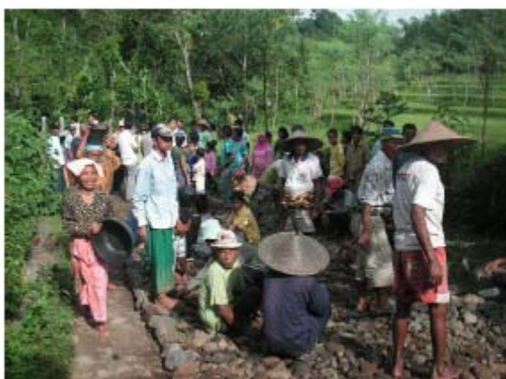
Collaborative Rehabilitation Works on Village Road by Local Community 16 (West Nusa Tenggara Province)
