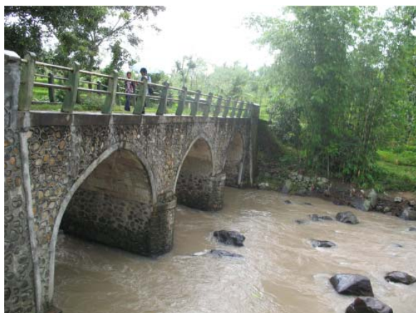
Bridge Constructed by Local Community Group (West Nusa Tenggara Province)
