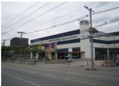
(a) Thailand Cultural Center Station
