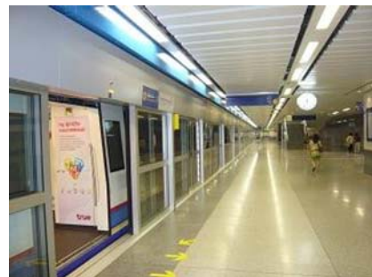
Figure 2: Door shields installed on platforms
