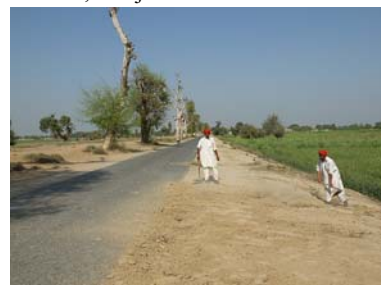
Fig. 3 Repair of road edge in Kabula, Punjab
