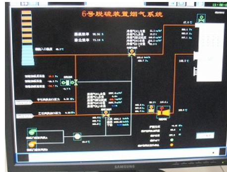
Figure 5: Exhaust gas desulfurizer monitor
