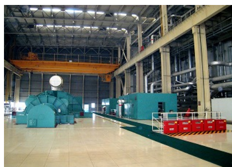
Interior of Jiujiang Thermal Power Plant Part III
