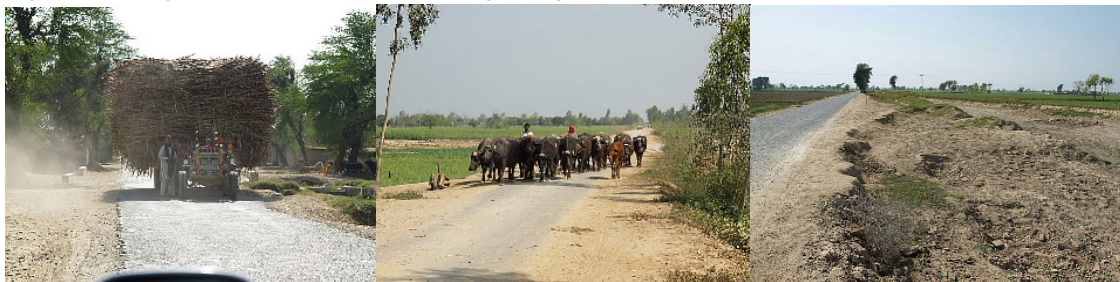
Fig.4 Crumbling of the bank due to overloading of sugar cane and to buffalos
