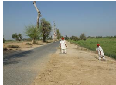
Fig. 3 Repair of road edge in Kabula, Punjab
