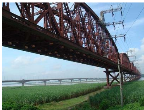
Hardinge Railway Bridge and Paksey Bridge
