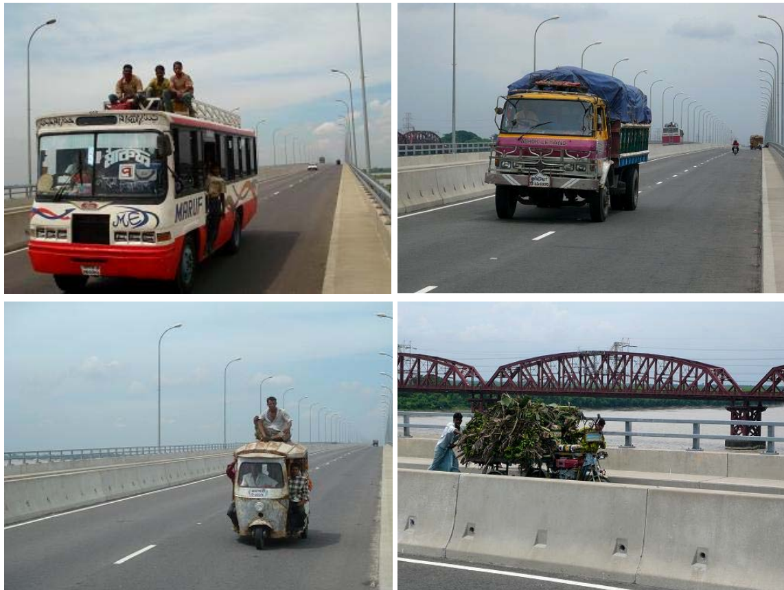
Various types of vehicles passing over Paksey Bridge: bus (upper left), truck (upper right), 3-wheeled taxi (lower left), light vehicle modified from motorcycle (lower right)
