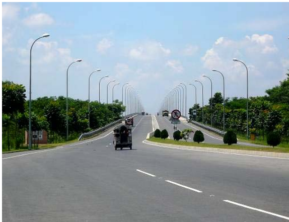
View of Paksey Bridge from the north side toll booth each side
