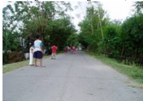
Figure 9: Paved levee (right bank of Agno River)
