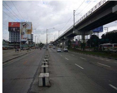
EDSA/Quezon Interchange Flyover along EDSA
