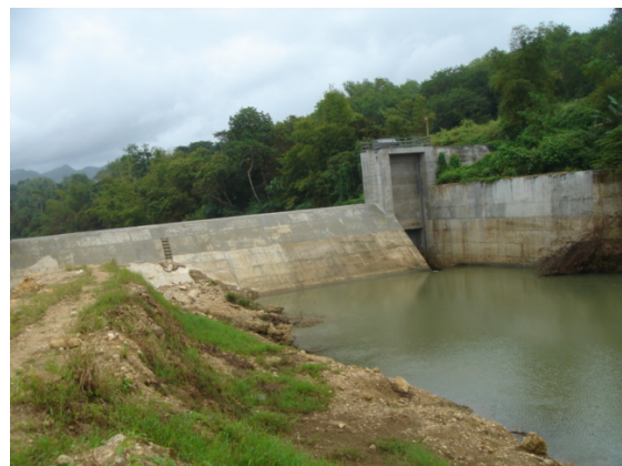
Hydro Power Facility constructed under EISCP2
