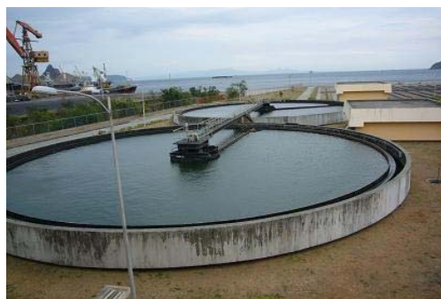
Sewage Treatment Plant in Bataan
