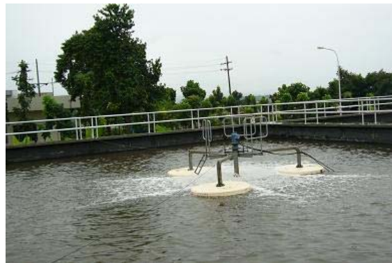
Sewage Treatment Plant in Mactan
