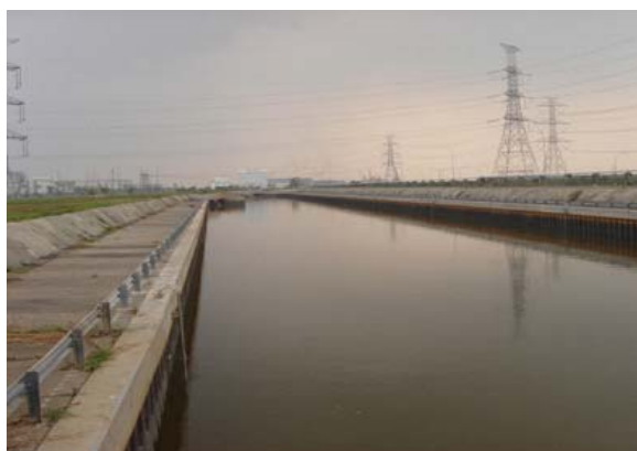
Cooling Water Channel
