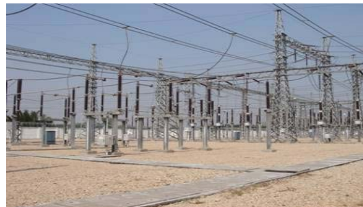
Nha Be Substation
