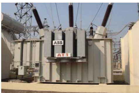
Bac Giang Substation
