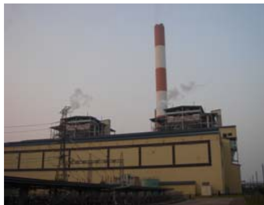
Pha Lai Thermal Power Plant
