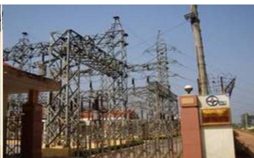
Soc Son Substation
