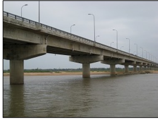
Ngon Son Bridge (Phu Yen Province)
