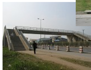
Additional output (frontage road and pedestrian bridge)
