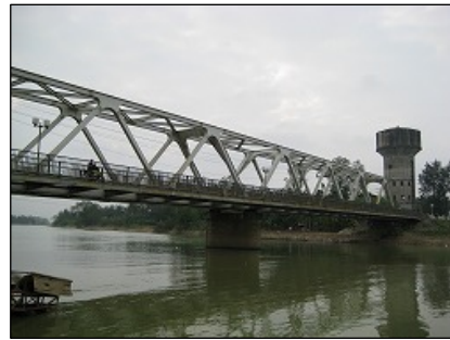
Gia Vien Railway Bridge (Hue)
