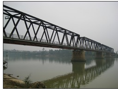
Cho Thuong Railway Bridge (Ha Tinh Province)
