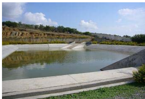
Treated sewage reservoir (Medenine)
