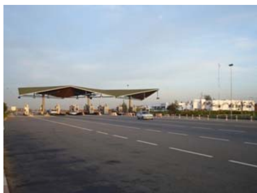
South Ring Road Tit Mellil Toll Station
