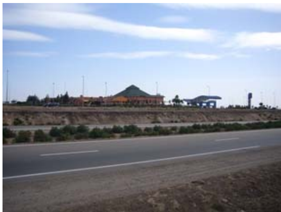
Casablanca-Settat Expressway Berrchide Service Area
