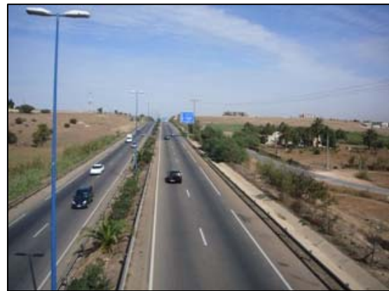
Starting point of the Casablanca-Settat Expressway
