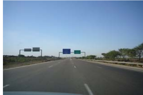
Starting point of South Ring Road
