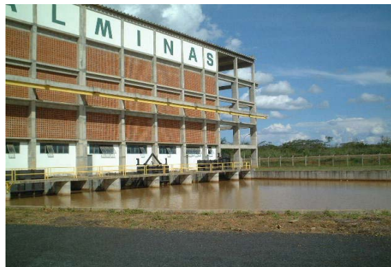
Figure 10: Jaiba 2 sluice gate
