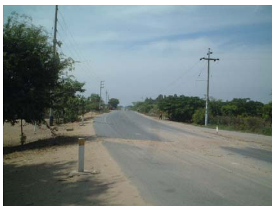
Illegal speed bumps set up by residents
