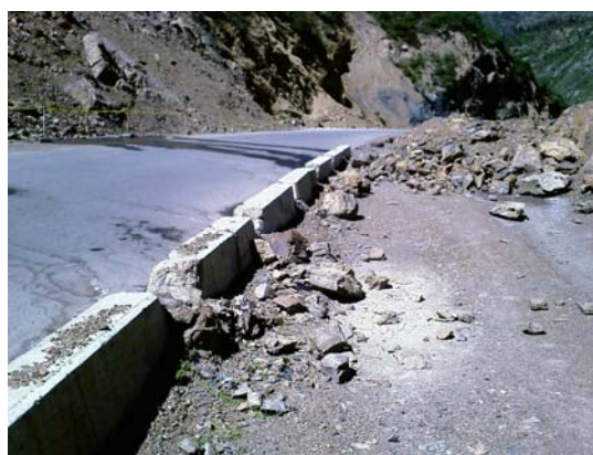
Roads damaged due to landslide
