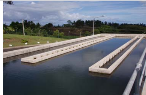
Buabua Water Treatment Plant
