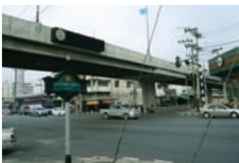
An overpass constructed
