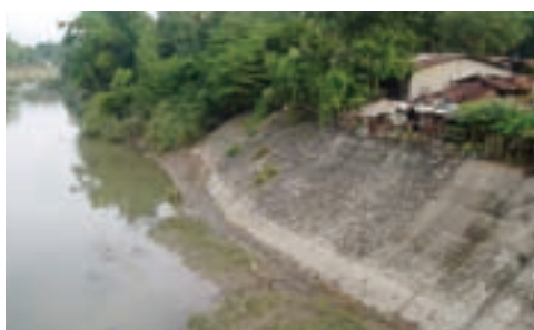
Bank revetment along the Sinocalan River
