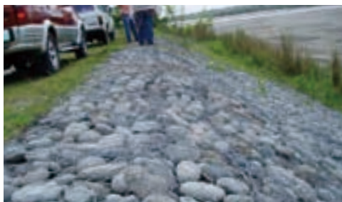
Rehabilitation of a levee on the right bank of the Tarlac River
