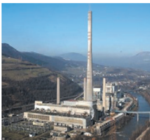
Kakanj Thermal Power Plant
