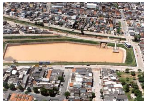
Figure 7: Rainwater Runoff Reduction Facilities (Flood Control Reservoirs)
