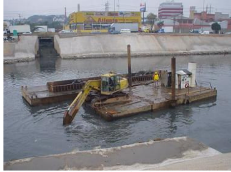
Figure 17: Work of Silt Removal
