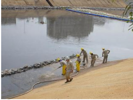
Figure 16: Work of Periodical Maintenance
