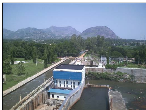
Small Hydroelectric Plant (State of Tamil Nadu)
