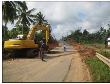
Ongoing road improvement work (at the 2-3 km south from Jepara)
