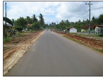
Ongoing road widening work (at the 2-3 km south from Jepara)
