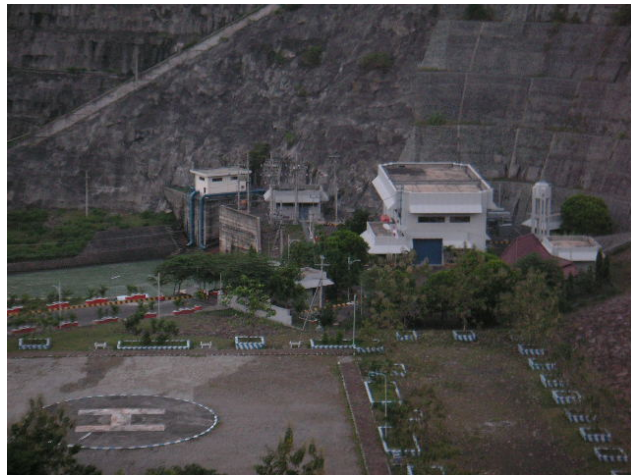
Distant view of Wonorejo Hydroelectric Power Plant
