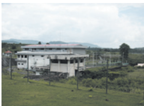
Bili-Bili Power Plant
