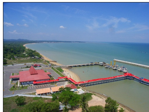
Ferry terminal constructed under this project (Muntok)
