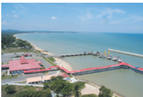
Ferry terminal constructed under this project (Muntok)
