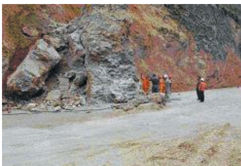
Rock Clearing works (Jauja-Tarma section, Junin Region)
