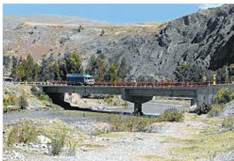
Bridge constructed under the project (Junin Region)
