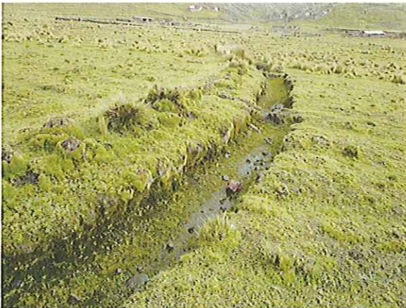
Infiltration Ditch at Highland Swamp
