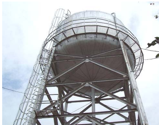
Elevated water tank
