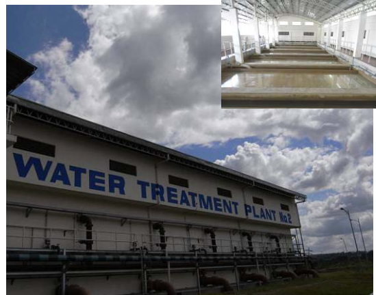
Water treatment facilities constructed under the Project (San Jose Del Monte City)
