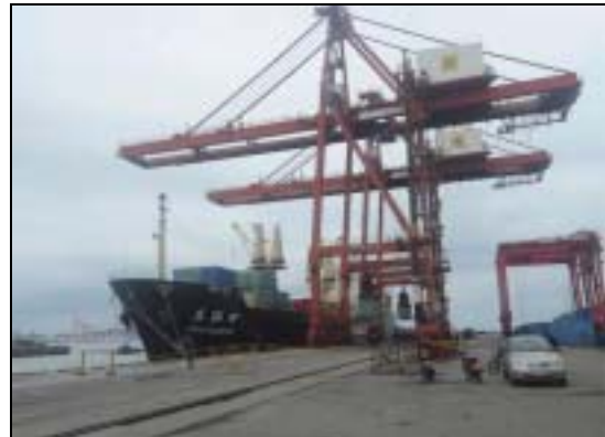
North Pier of the Port of Colombo
