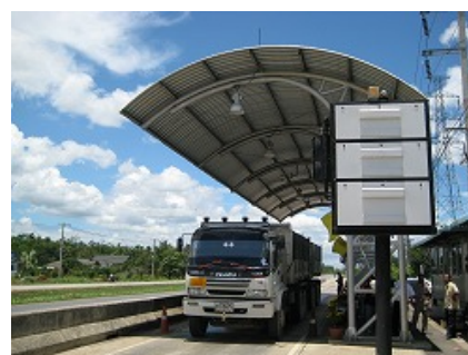
Weighting Stations installed near Don Sak Junction on NH401
