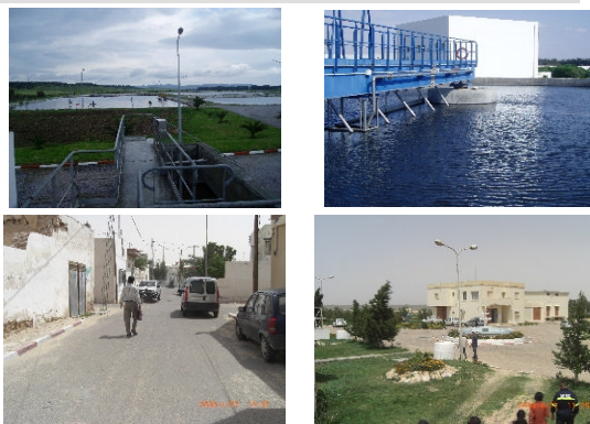
(Clockwise from upper left) Zriba Sewage Treatment Plant, Sfax North Sewage Treatment Plant, Kebili Sewage Treatment Plant, Douz residential area
