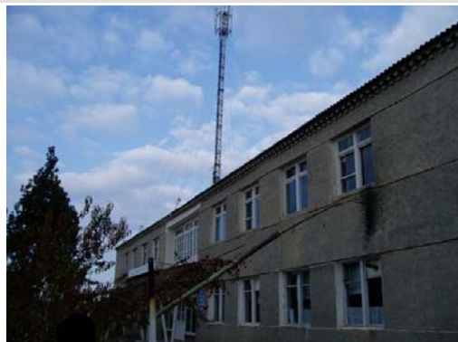
One of the Backbone Transmission System stations operated by Bukhara Telecom
